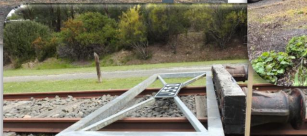
GATE READY TO BE INSTALLED AND PAINTED
