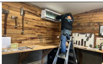
Installation of a new air conditioner in the Platform and Goods Shed, along with storage modifications in preparation for a television screen on the side wall
